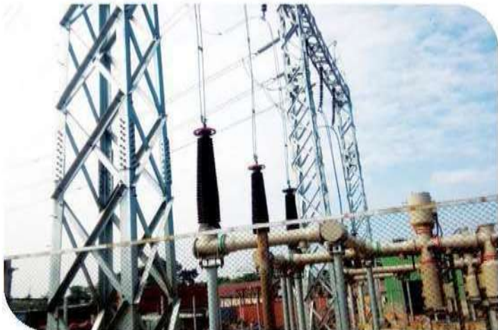
Kushiara Power Plant - a project by Pubali Bank Limited Principal Branch, Dhaka
